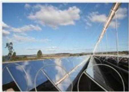
These are several mirrors which have been arranged and sharing the same receiver. Fresnel reflectors have the advantage of reduced tracking mechanism complexity. They are also stationary absorbers.
