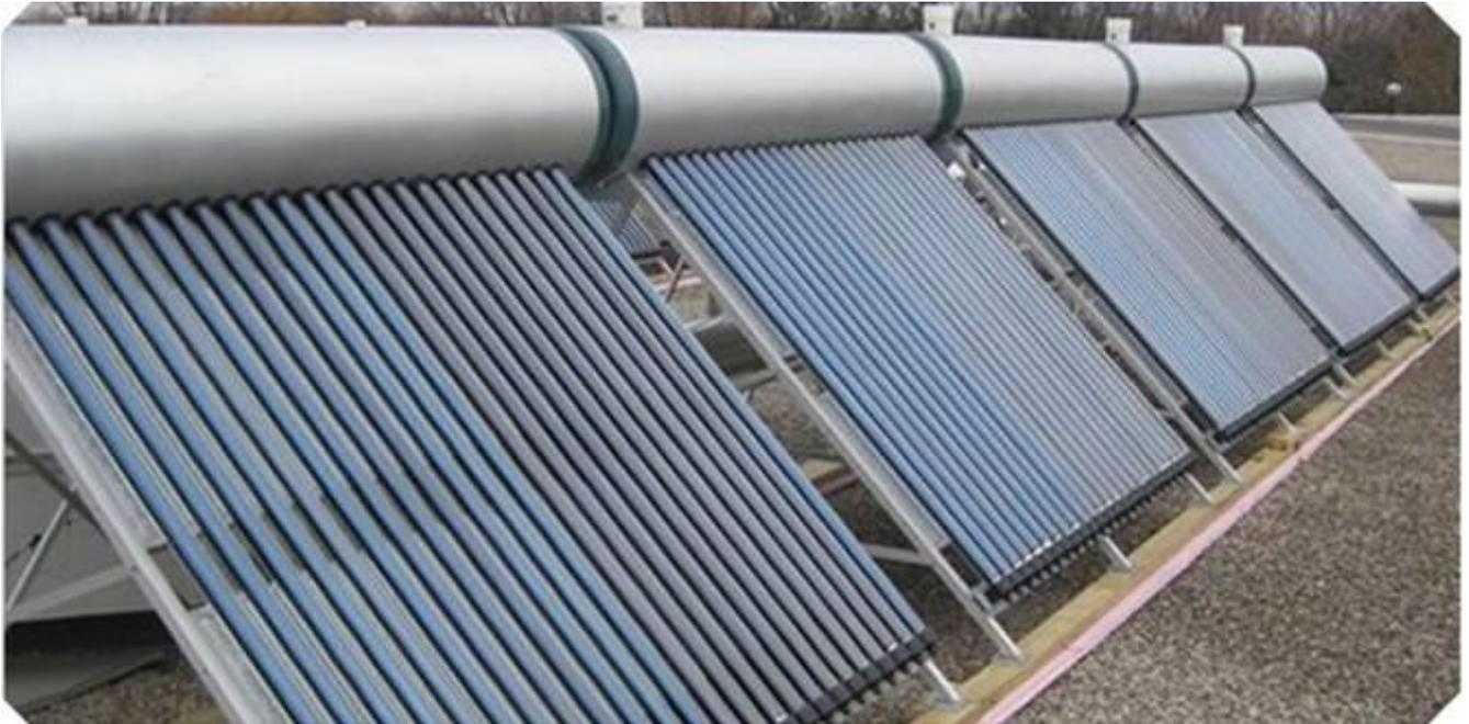
Fig. 6 Glass-Glass Evacuated Tubes Absorber
